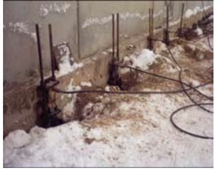
Torealign beam, 38 CHANCE® helical tieback anchors were installed between Atlas Resistance® piers.
