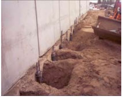
With wall elevation restored and beam straightened, pier holes were filled to final grade.
