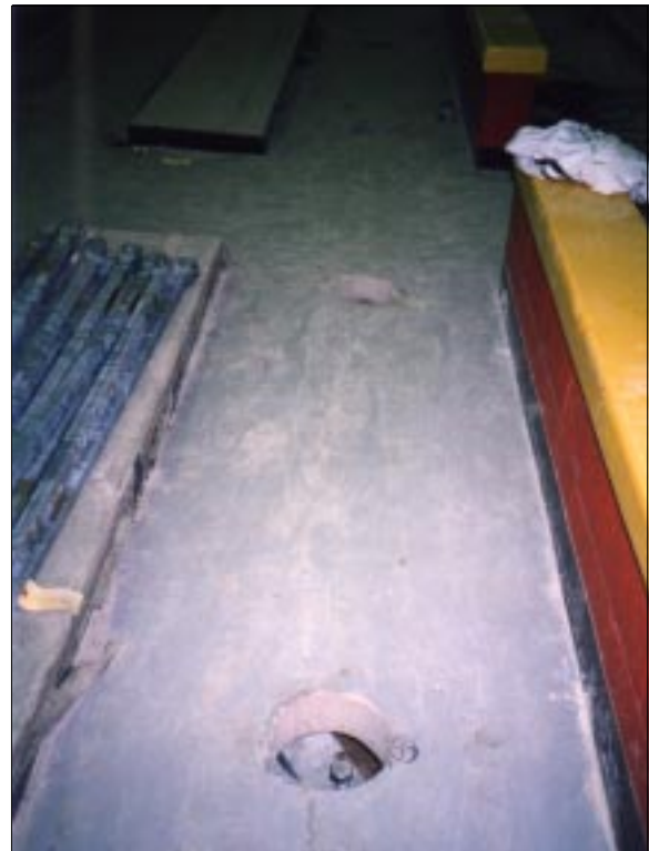
Slab-leveling anchor being installed and bracket bolt visible through core which was refilled after final adjustment.
