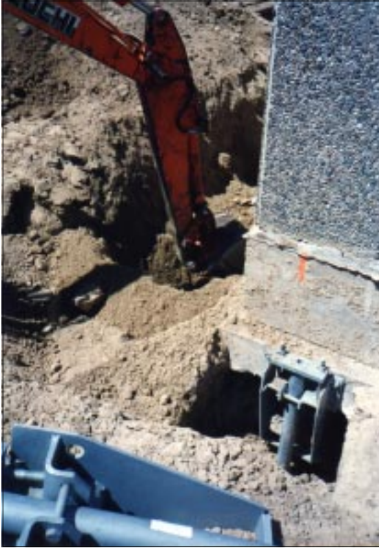
Heavy-Duty underpinning brackets installed outside and inside perimeter of foundation.
