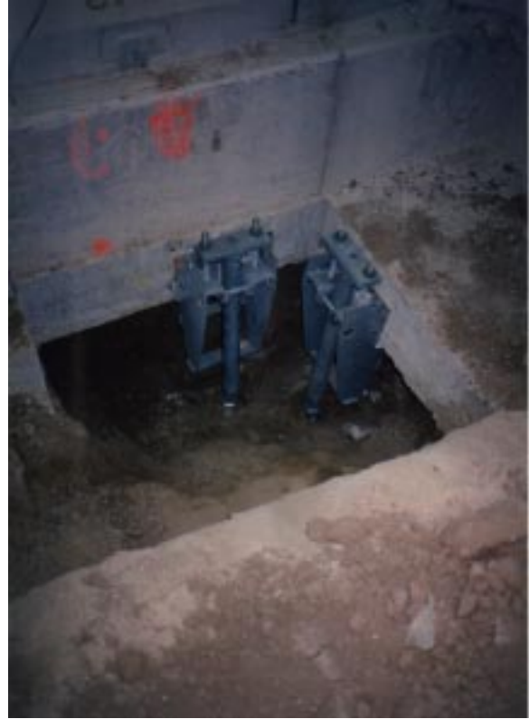
Heavy-Duty underpinning brackets installed outside and inside perimeter of foundation.
