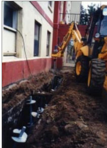
fit under and bolt to the side of the foundation. The load of the structure is transferred from the foundation to the anchor via the bracket. For new construction, a T-shaped piece is fitted over the end of the anchor. Reinforcing steel is then tied or welded to the bracket before being cast into a concrete grade beam.
