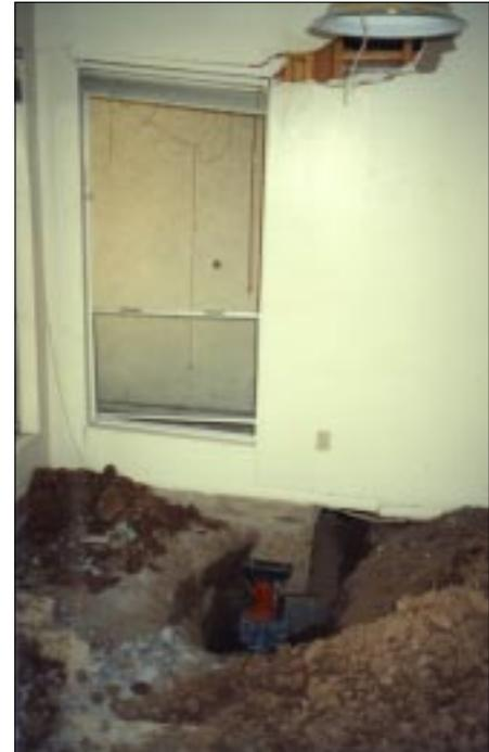
ing installation torque, the capacity of a screw anchor can be determined. A known safety factor can thus be established.
