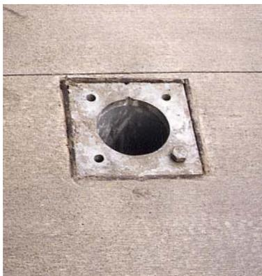
*Foundation base is flush with the concrete walk.*
