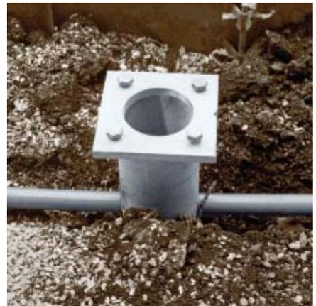
*Conduit runs through the cable entry slots provided on each foundation.*
