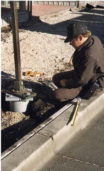
*The foundation type used by the city is 5' in length with a 1" x 12" base plate. Bolt circle is 11". The cableway size is 2 1/2" x 12". The cableway distance is 12" from the base plate. 1" x 2 1/2" hex-head bolts are used to mount the standard to the foundation. The helix is 14" in diameter. Catalog No. is C11242NG4TK.*
