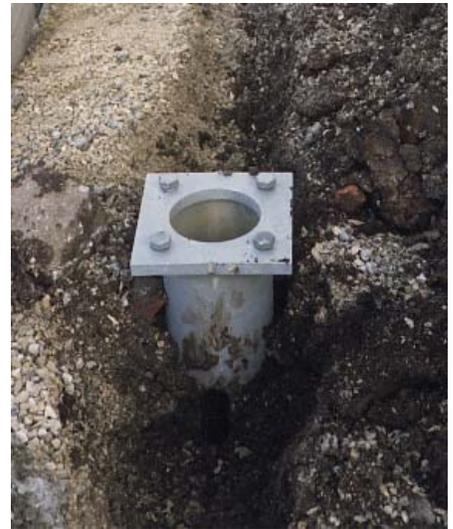
*With Chance power-installed area-lighting foundations, the users have a versatile alternative to using cast-in-place or precast concrete foundations.*
