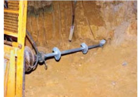
termination. A 4 x 5 ft. grid was determined for use on this 100 x 50 x 21 ft. excavation. Boring logs showed the screw anchors were installed in firm and very firm, silty coarse-to-fine sand with Standard Penetration Test results typically from 10 to 20 blows per foot. Preloads of 20,000 lb. tension were selected for one to two tests per site.
