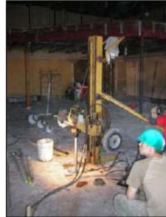
Hand held units for interior works have similar capacity. However they can be carried in sections and snapped together in restricted areas. That feature allows use in such tight spaces as, closets, small bathrooms and crawlspaces.
