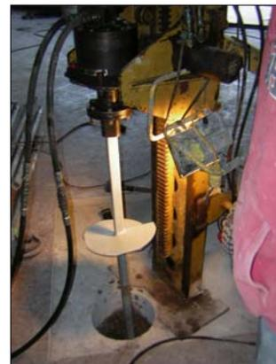
Installation torques over the terminal three feet of insertion reached 5500 ft/ lbs
